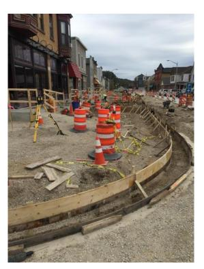
Crews worked last week to frame the curb and sidewalks along the west side of Main Street. This work really helps display the future shape of west side of the street. The upcoming week will include placing concrete pavement south of Washington Street. Crews will also be completing the ADA ramps along the sidewalk on the west side of the street.
