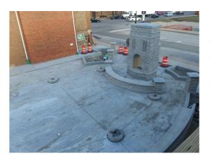
Construction crews have made great progress at Historic Village Hall. The concrete has been installed creating the base for new brick work that will be added once temperatures increase. The new outdoor fireplace has also taken shape. This feature will be completed in the coming weeks when the remaining top section is added.
