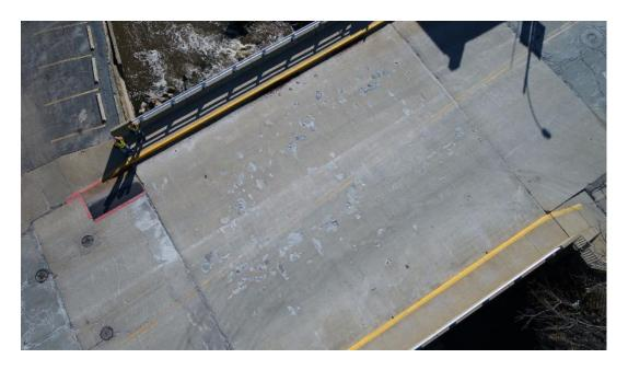
Crews will remove the bridge deck (roadway portion of the bridge) surface throughout the week. The removal process will include saw work on Wednesday as crews prepare sections of the structure for removal. Please note that the saw work may cause some noise disruption and dust in the downtown on Wednesday.
