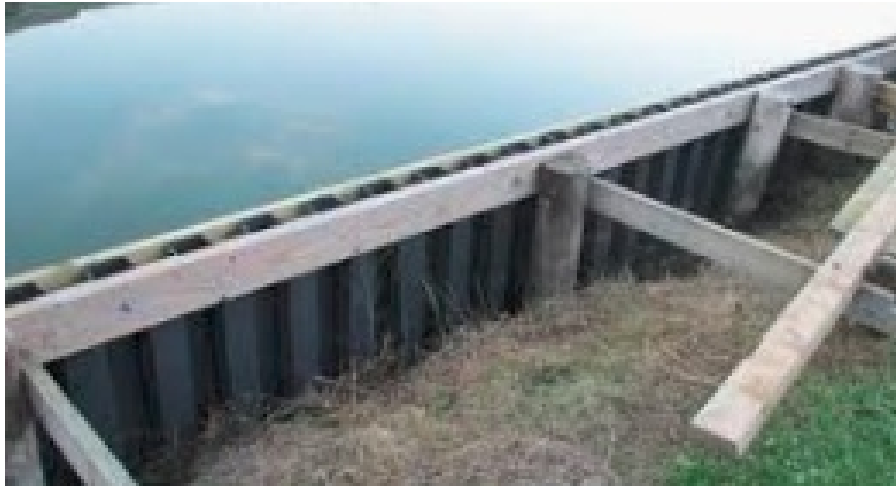
Sample image of sheet piles used on a bridge construction project.
