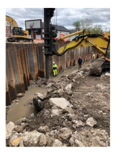
Crews will continue drilling the shaft foundations for the bridge over Crystal Creek this week. Crews need to drill 30 holes for the foundation before the next phase of bridge construction can begin.
