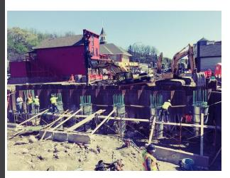
This week, drilling will continue for the shaft foundations needed for the bridge over Crystal Creek. This work is labor intensive, as crews are drilling 30 holes for the foundation. Construction of the bridge is anticipated to be completed this summer. Once the bridge structure is finished, a decorative archway will be added welcoming residents and visitors to Old Town.
