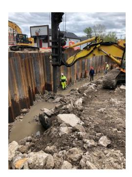
Friday's favorable weather allowed crews to finally begin drilling the 30 holes needed for the bridge foundation. These deep holes or shafts will be used to support the bridge structure. Work on the bridge will continue as weather permits.
