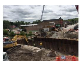
Construction of concrete retaining walls and abutments for the bridge will continue this week. The abutments will connect the surface of the bridge to the ground and help support the weight of the roadway over the bridge.
