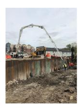
Construction of the bridge continues with progress being made on the supporting structures. Crews completed the north section bridge concrete retaining walls and abutments this past week. Focus will now shift to pouring the concrete for the southwest retaining walls. Once that work is completed the abutments for the south section of the bridge will be constructed.
