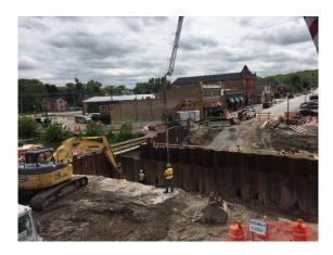
While the wet spring has not been ideal, crews have continued to work and installed the center pier support for the bridge structure and finished drilling the shaft foundations on the south side. Crews will begin the same drilling process for the shaft supports on the north side. The drilling has also been completed on the shafts for the north abutments or ends of the bridge.
