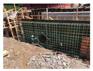
Progress continues to be made on installing the substructure of the bridge. This week, crews will continue the process of pouring concrete and forming the south abutments for the bridge.
