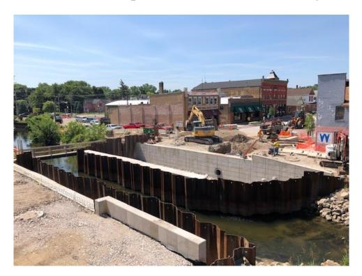
This past week, the work zone area around the bridge was back filled. The work zone area had been previously excavated to allow crews to work at the base of the creek during the construction of the new bridge substructure. Now that this work is complete the area was filled with construction material that will eventually support the new roadway on either side of the bridge.
