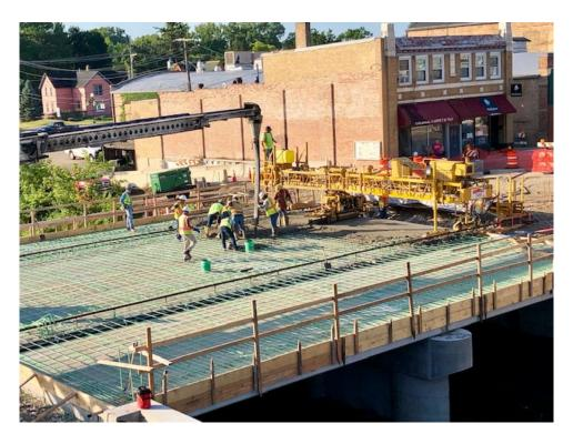
Construction crews have completed pouring the first layer of concrete for the bridge deck over Crystal Creek. The second layer of concrete will be poured this week to create the curbs and pedestrian sidewalks. It takes several days for concrete to fully cure or dry. During this time, crews will begin work on the water main infrastructure on the north side of the bridge.
