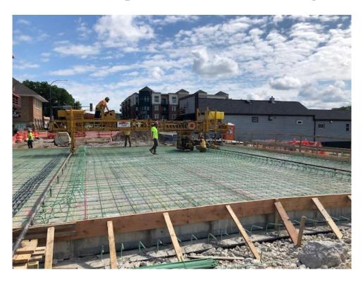
The construction team has been busy preparing the bridge structure for concrete. This included installing the electrical conduit and rebar into the structure of the bridge, pictured above.
