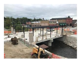
Progress continues on the bridge over Crystal Creek. This week, crews will be installing the handrails over the bridge and installing lights in the pergola. These features will help create a safe and inviting walkways for pedestrians. Crews will also begin to prepare the area for new sidewalk concrete that will be installed on both sides of the bridge.
