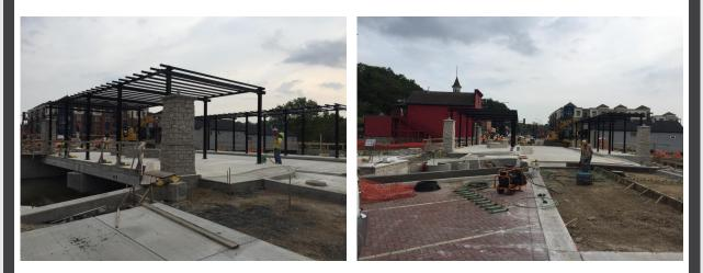
Crews are focused on transforming the section of Main Street between the bridge and Algonquin Road. New brick pavers will be installed on the west side of Main Street along with new curbs and gutters. The roadway in this section is also being graded in preparation for new pavement to create a safe and smooth entrance into Old Town.
