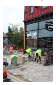
New brick pavers have been installed along the north section of Main Street between the bridge and Algonquin Road. The pavers create the same charm and character that was created south of the bridge along Main Street.
