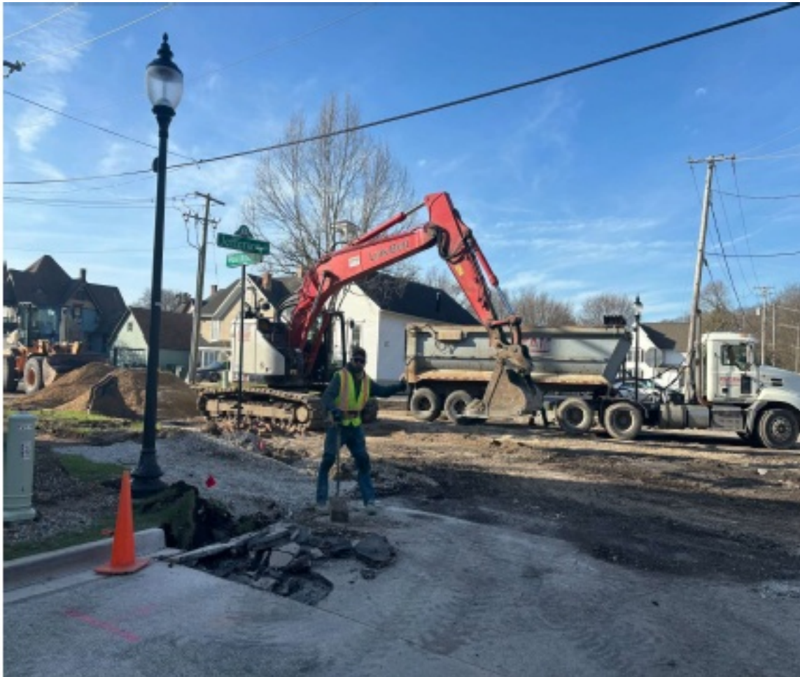
Asphalt removal on West Washington Street
