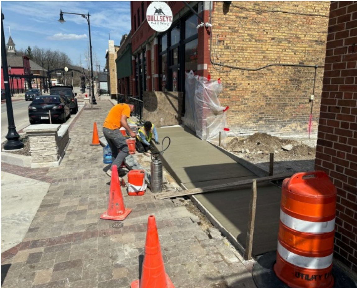
Finishing the new ADA ramp at Bullseye Pub
