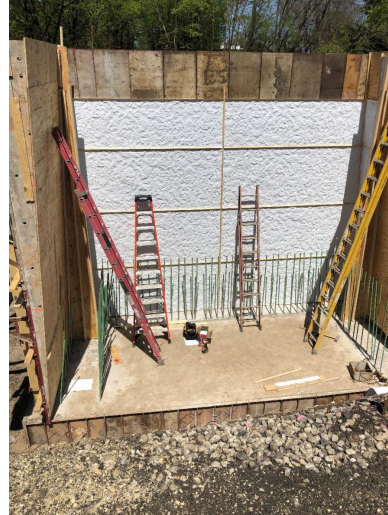
East abutment wall form work with liner
