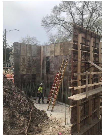
Abutment wall taking shape
