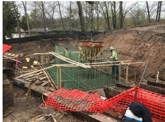
North abutment wall foundation
