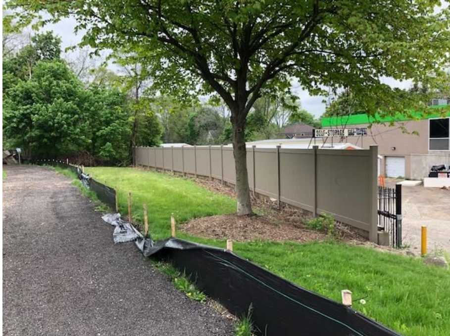
New fencing installation
