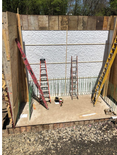
East abutment wall form work with liner
