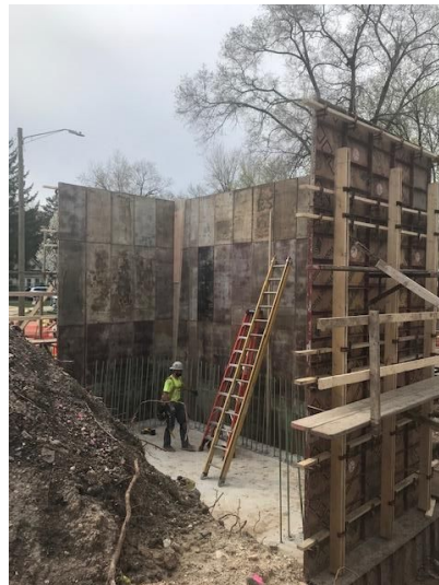
Abutment wall taking shape
