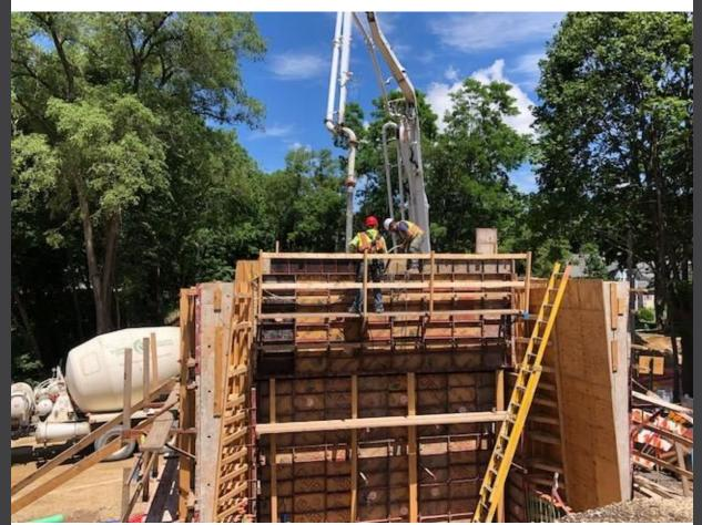
Last week, crews placed the concrete for the bridge abutments that will hold the new pedestrian bridge.
