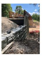
This week, crews continued installing the retaining walls, adding drainage and replacing (backfilling) the soil that was disturbed around the abutment walls.
