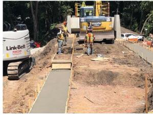
This week, crews continued installing the retaining walls, adding drainage and replacing the soil that was disturbed around the abutment walls. They also worked on grading the connection to the Prairie Trail.
