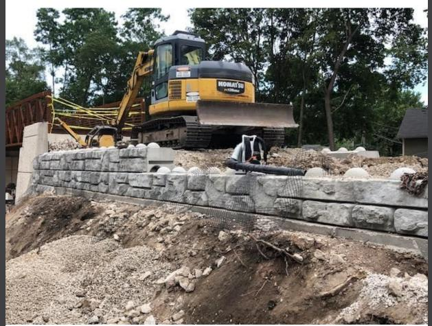
This week, crews continued installing the concrete block retaining walls and creating a level connection to the Prairie Trail. Next week, crews will continue these efforts and will place the bridge surface reinforcement.
