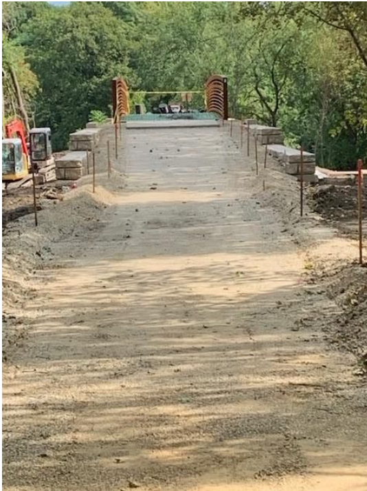
Regrading the connection to the Trail
