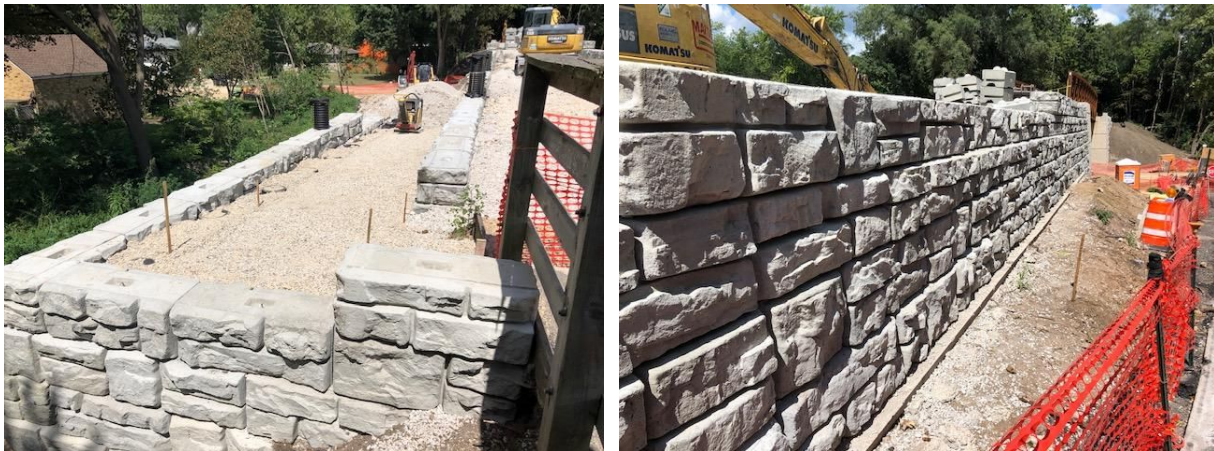
Concrete block retaining walls
