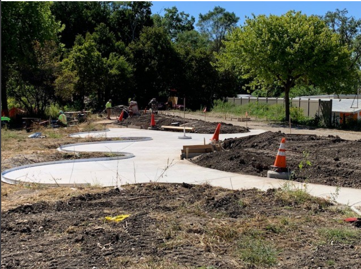
Paving for new pedestrian amenities
