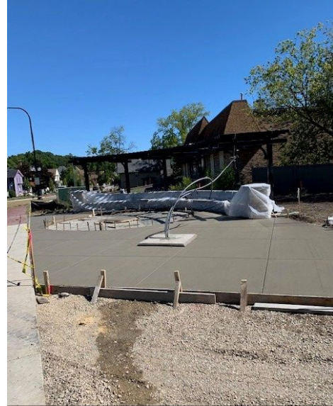
Placing the concrete base
