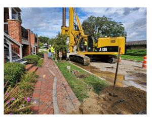
Last week, several dewatering wells were installed in the section of roadway north of Algonquin Road with the remaining wells expected to be installed today and fully operational.
