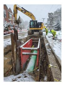
Last week, crews braved inclement weather to continue with the installation of the mainline sanitary sewer on North Harrison Street.
