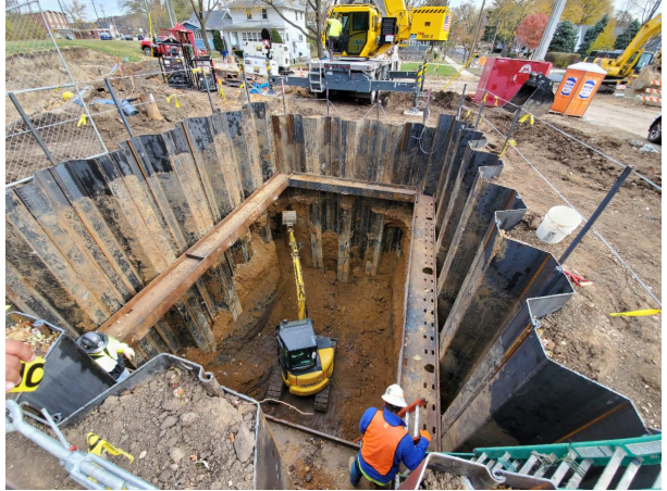
Lift station construction
