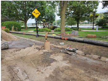
Photos of similar dewatering well installation
