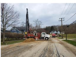
De-watering wells will also be installed near the intersection of Algonquin Road and Harrison Street over the course of this week. These temporary wells will lower the ground water elevation and keep trenches dry, allowing the utility work to occur. It is anticipated that Tuesday and possibly Wednesday the southbound land of South Harrison Street will be closed between Front Street and Algonquin Road for the dewatering wells installation.
