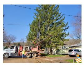
temporary de-watering wells along La Fox River Drive in preparation for the new sanitary sewer. Due to the location of the existing underground utilities several of these wells were installed within the sidewalk along the west side of La Fox River Drive. Pedestrians are urged to use the sidewalk along the east side of La Fox River Drive as several sections of the sidewalk are closed along the west side.
