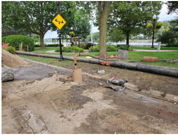
Photos of similar dewatering well installation
