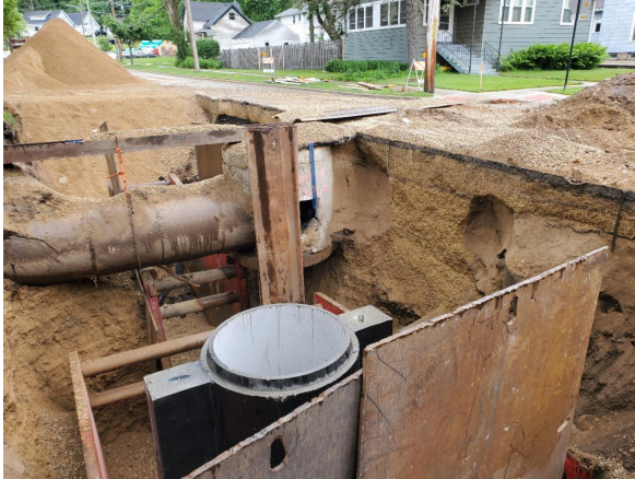
Sanitary sewer installation, road patching and concrete base course placement
