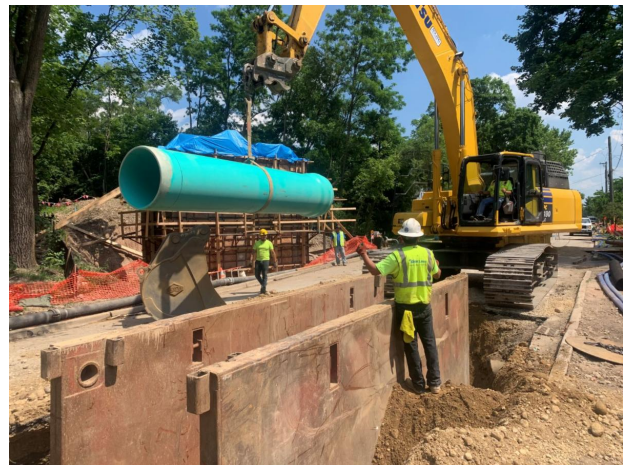
Sewer installation
