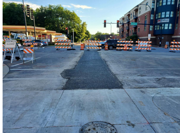
Main Street patching
