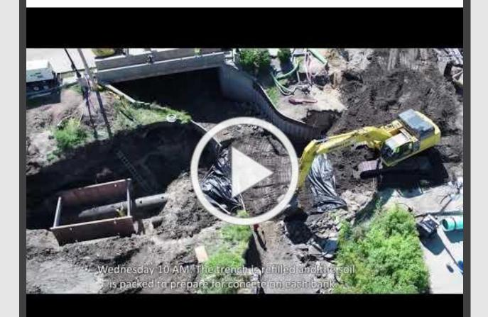
It only took **one week** for crews to finish installing the sewer and water pipes under Crystal Creek. Did we mention that the construction team worked day and night and literally had to move the creek, building dams and pumping the water (with by-pass equipment) around the work zone? Check out the <u>drone video</u> of this major infrastructure project!
