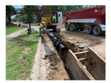
This week, crews began transferring the sanitary service laterals (or pipes) to the new sewer and the water services to the new water main along La Fox River Drive.
