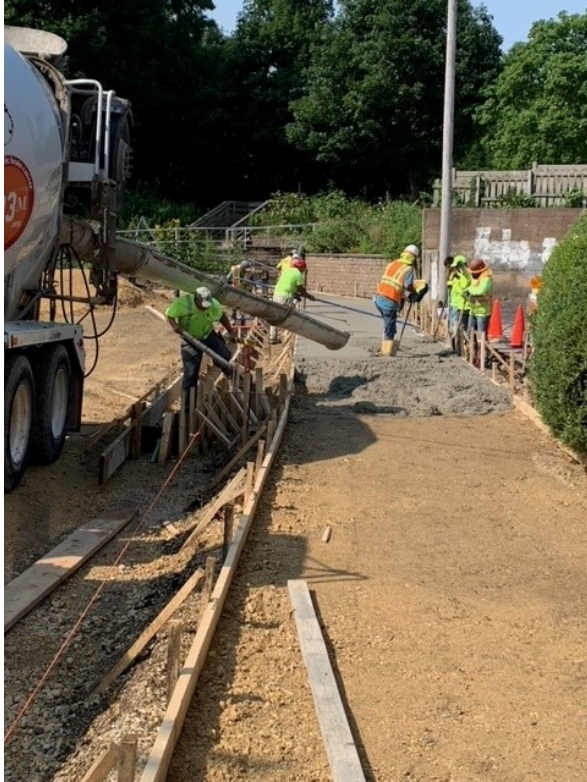
Pouring concrete for sidewalk
