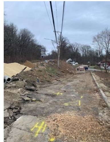
Clearing for multi-use path
