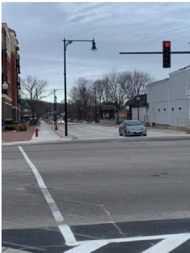
N Harrison Street reopened to two way traffic
