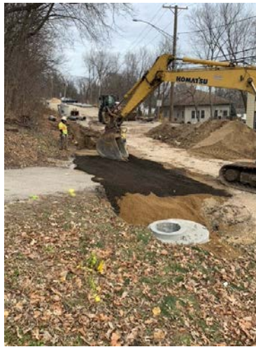
Stormsewer installation
