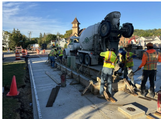
Placing concrete on Harrison Street
