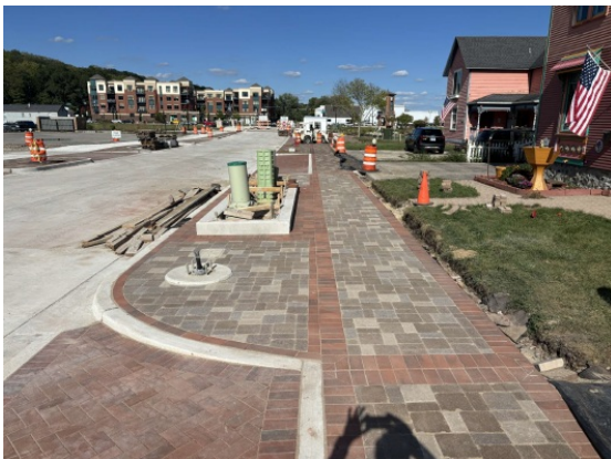
Brick paver installation on Harrison Street
